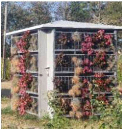
a) Western and Southern Façades
